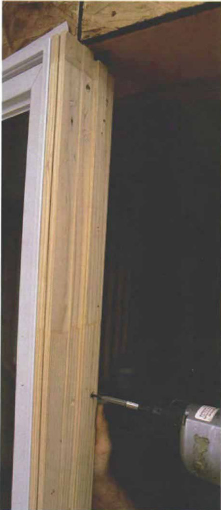
Fastening a spacer. A wedge-shaped pine spacer screwed to the window frame angles the windows to give the unit its bowed shape.
