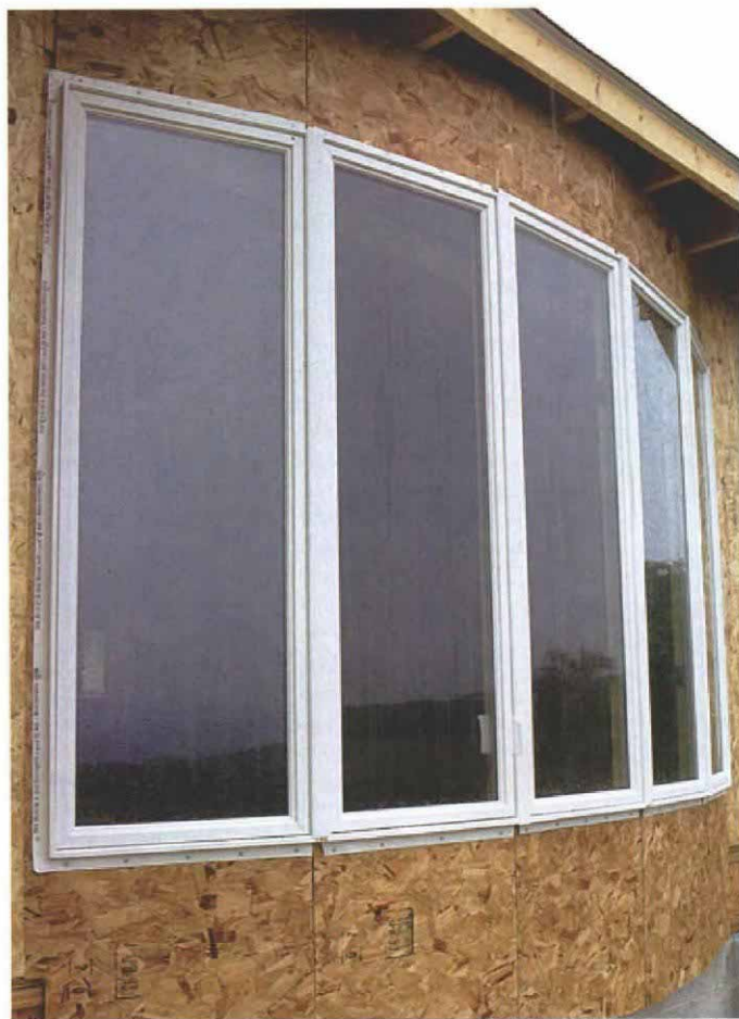
Windows from floor to ceiling. This 6-ft., high by 10-ft., wide Andersen walk-out bow window comprises five standard casement windows joined with wedge-shaped spacers. The unit projects 14 in. from the wall plane and is supported by cantilevered wood I-beam floor joists.
